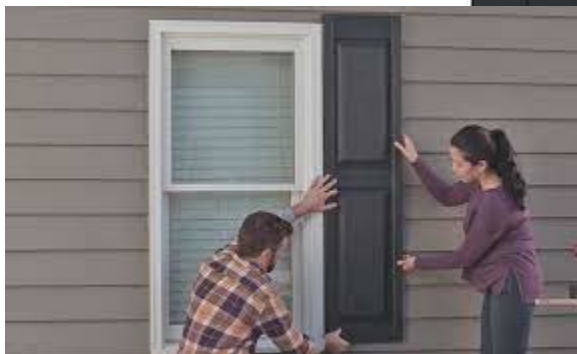
Installed onto siding
